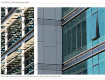
South Facade showing fixed fins and light shelves - Photo Credit: Photographs ©2012 Bruce Damonte. All rights reserved.
