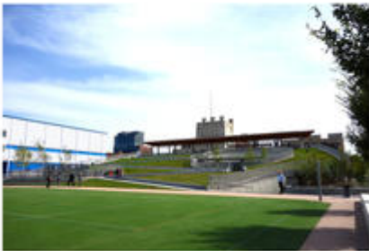
Building from sports field - Photo Credit: Kiss + Cathcart, Architects
